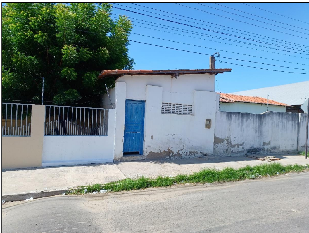
Figura 13 – Booster 1 (Booster Pêgas)
